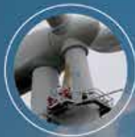
Nacelle and Blade Inspection & Cleaning
